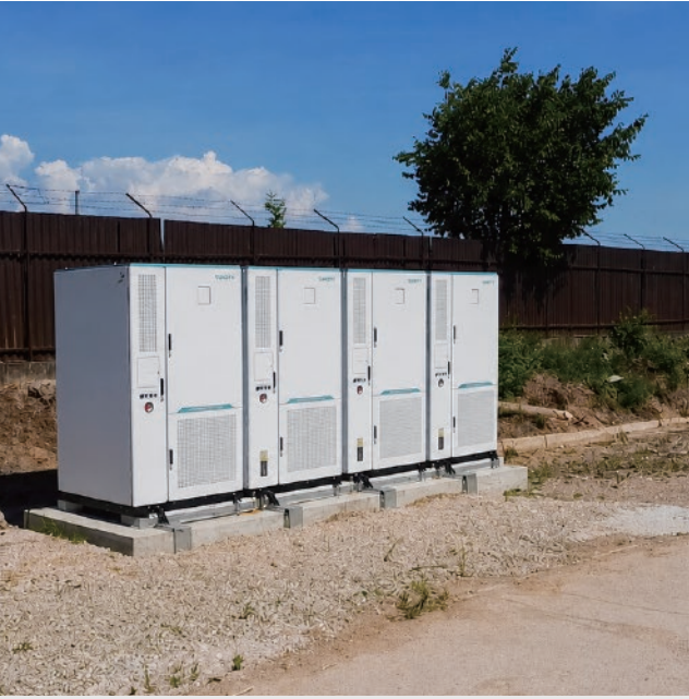
Petrich, Bulgaria Battery capacity: 932 kWh
